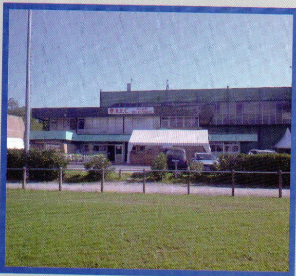
Le Club house - Terrasse restaurant
